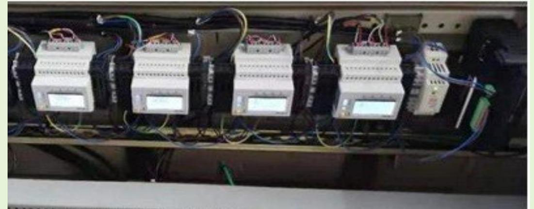
**Project Overview:** Client buy Acrel ADW200-MTL multi-loop leakage current monitoring meter, with AKH-0.66/L leakage current transformer, to connect with client' own gateway and software monitoring system.
