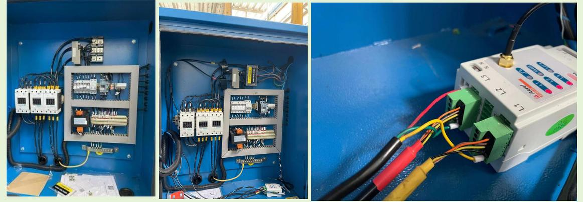
Project Overview: Client buy Acrel AEW100 LORA 868MHz wireless consumption monitoring meter, to connect with their own gateway and software monitoring system. Then the custom demand was put forward to add 5V output terminals to supply power to the external microcontroller.
